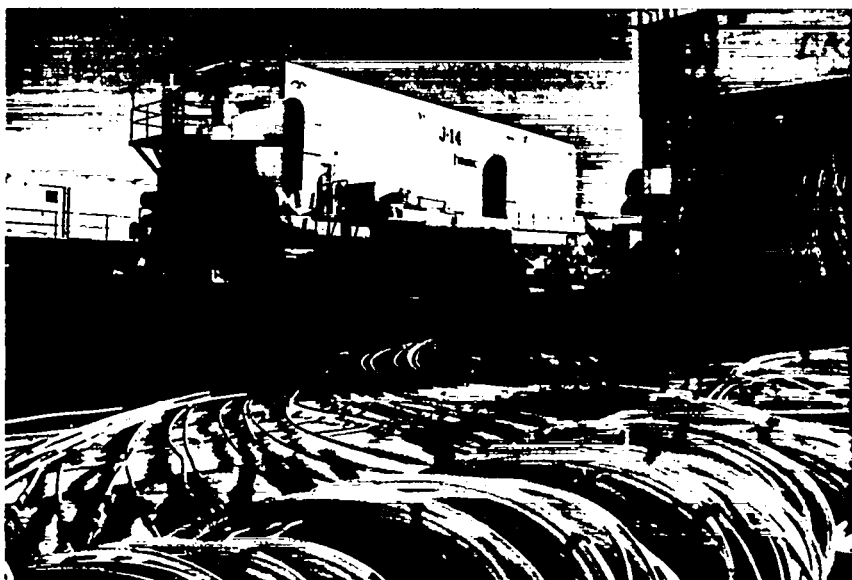
Numerous cables connect instruments on the rack with above-ground recording stations.
